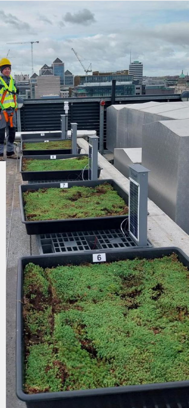
↑ Green roof trial 1WML
