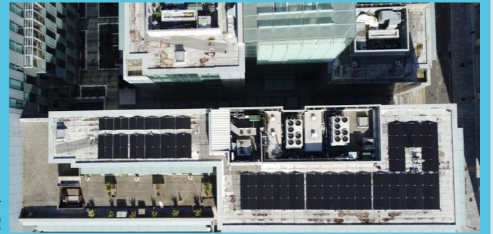
Solar PV panels Central Quay
